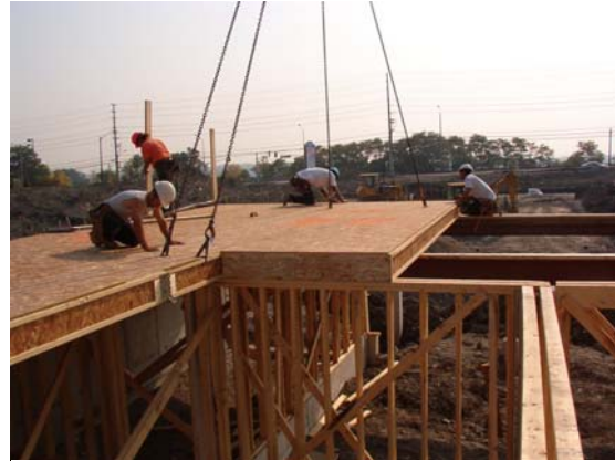
All materials, including joists, rim board, beams and floor panels, are marked and can be installed quickly and easily according to a placement plan developed using iLevel® Javelin® software.
