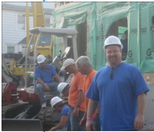
Tom Pivovar helps with the installation of Daikin's donated VRV-S system.
